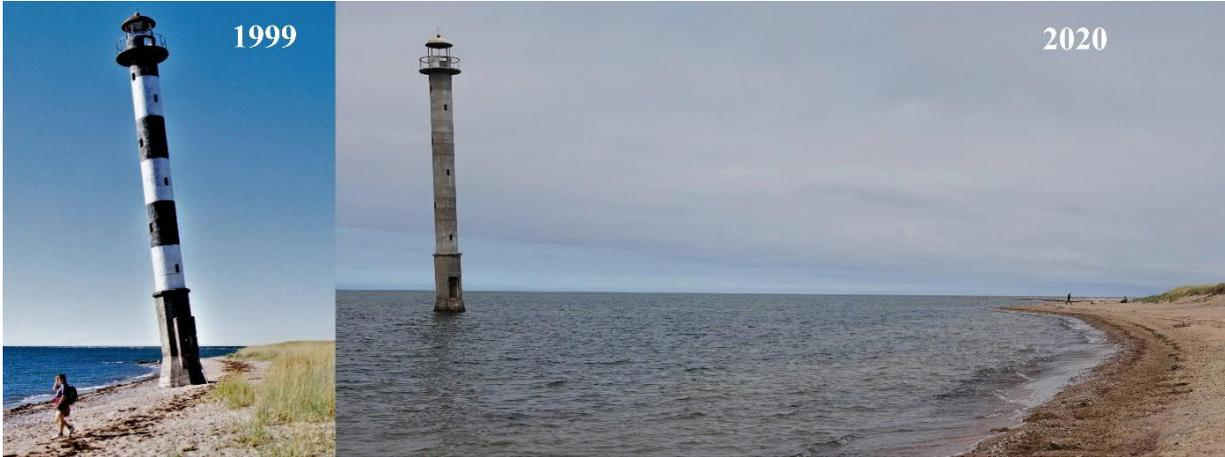
**Figure S1.** Location of Kiipsaare lighthouse (height 25 m) in relation to the shoreline in 1999 and 2020 (photos: Ü. Suursaar).
