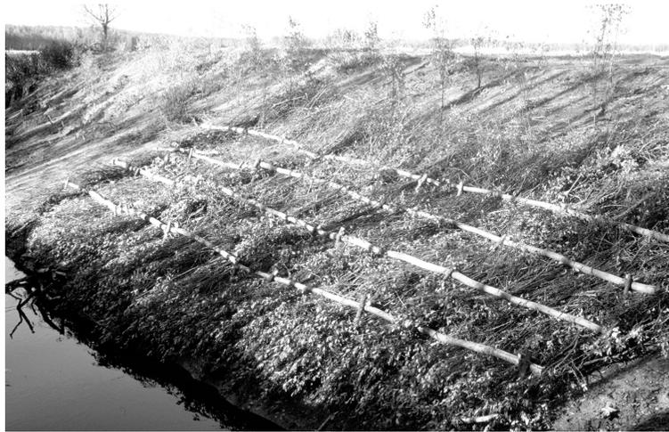
**Fig. 3.** Example of applying brush mattresses in reach P2 of the Pääntäneenjoki.
