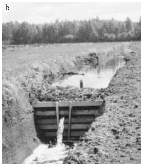
Fig. 2. Overview of water treatment structures. (a) Schematic overview of constructed floodplain, peak runoff control structure and sedimentation pond. (b) Peak runoff control structure during flooding event in August 1996. (c) Peak runoff control during snowmelt.
